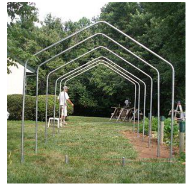
Fig 3.1 Bow Installation
